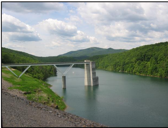
Figure 13. Gathright Dam intake tower (USACE photo).
